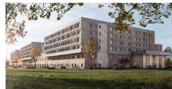
2023 Cluj Regional Emergency Hospital
