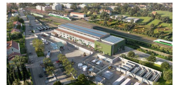
2025 Hydrogen Production and Refueling Station
